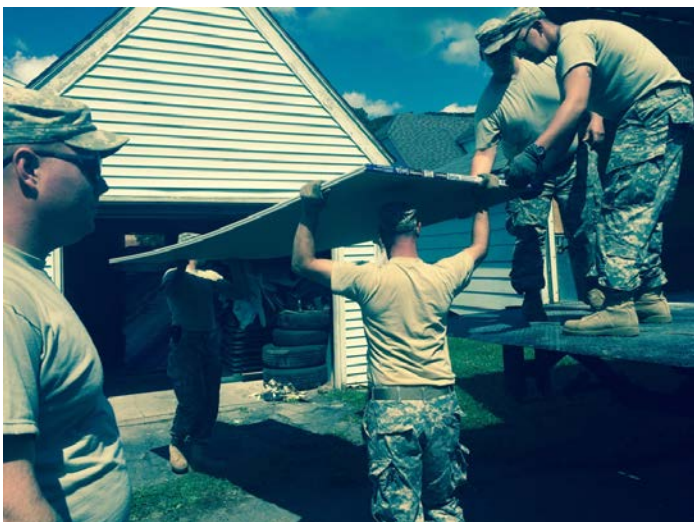
Drywall delivery to Webster County 2016
